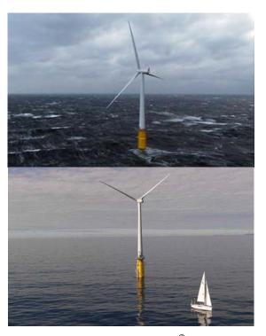
Figure 5.2.2 Left: Hywind concept, Siemens 2.3 MW-82 turbine on a 65 m base <sup>©</sup>Statoil .Right: Turbine at site in various wind conditions
