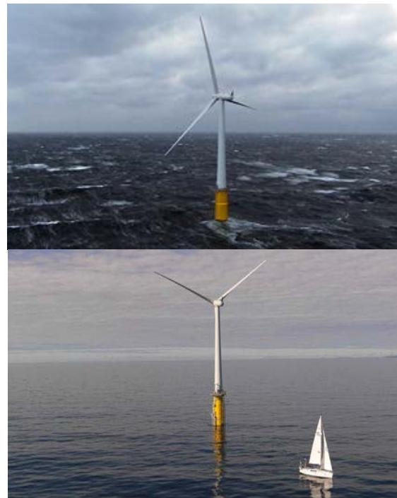
Figure 5.2.2 Left: Hywind concept , Siemens 2.3 MW-82 turbine on a 65 m base ©Statoil . Right: Turbine at site in various wind conditions
