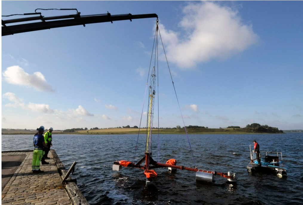
Figure 63 Deployment of the demonstrator by truck crane to the sea next to the pier
